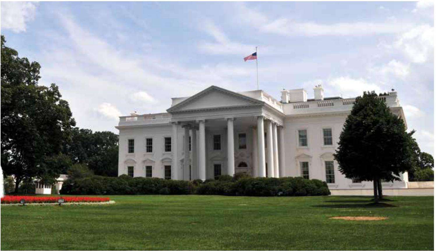
Atlas Provided FAP42Ts for the White House Press Room
